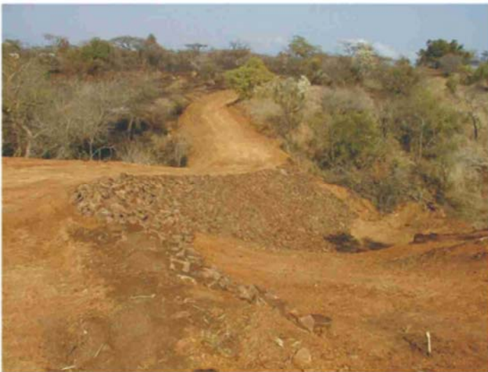
Example of bush clearing
