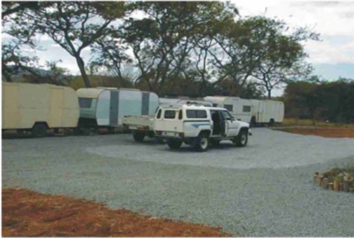
Example of site offices
