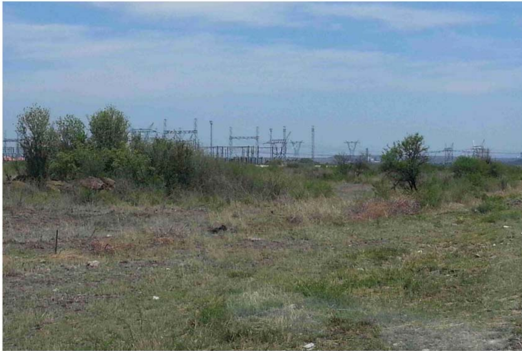
VIEW A: VIEW TOWARDS EXISTING MARANG SUBSTATION
